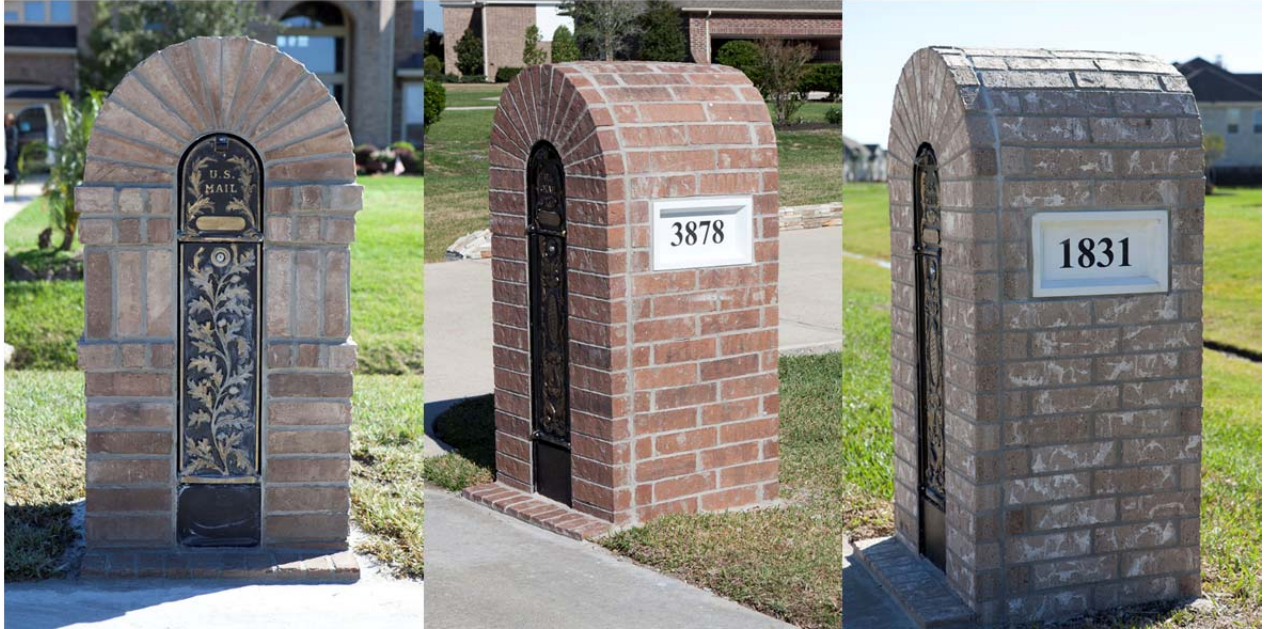
Figure 1: Locking Brick Enclosure Mailboxes. Simple arch design with brick matching home is the accepted standard. Street numbers in cast white block the same as house address block.
